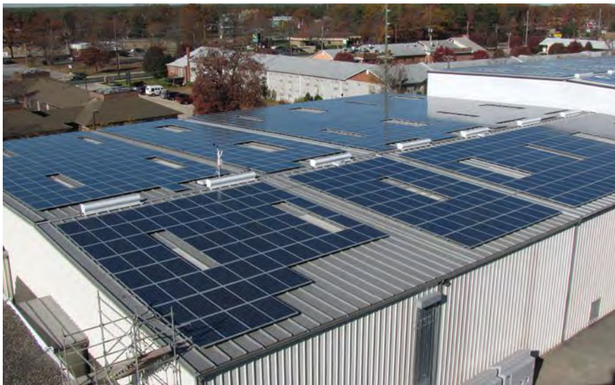
Solar panels on Espoma’s facilities occupy roughly a square acre and power all its operations.
