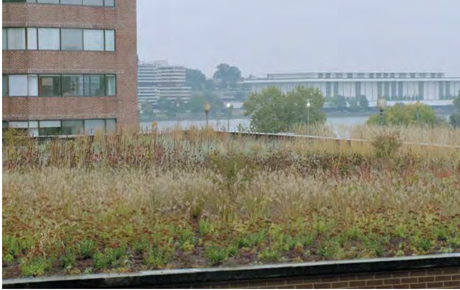
Above left: Designed by Oehme, Van Sweden Associates, this semi-intensive green roof at the Pepco Building in Washington, D.C., features ornamental grasses, forbs, and sedums. Above, right: Biodegradable mesh helps sedums take root in an extensive green roof garden.
