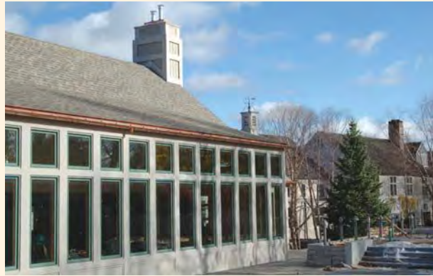
Large windows provide the new center with plenty of light.
