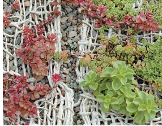
Above left: Designed by Oehme, Van Sweden Associates, this semi-intensive green roof at the Pepco Building in Washington, D.C., features ornamental grasses, forbs, and sedums. Above, right: Biodegradable mesh helps sedums take root in an extensive green roof garden.
