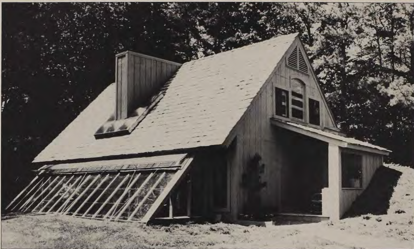
The dug foundation of this greenhouse (pictured from the inside on page 30) provides extra insulation from both heat and cold.
