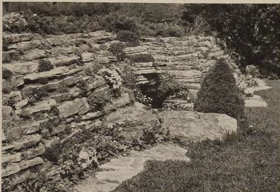
Dry wall just after building
