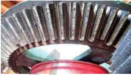
Iron turbine wheel with teeth made of service tree wood in the hydro-electric power station near Tournus, France.
