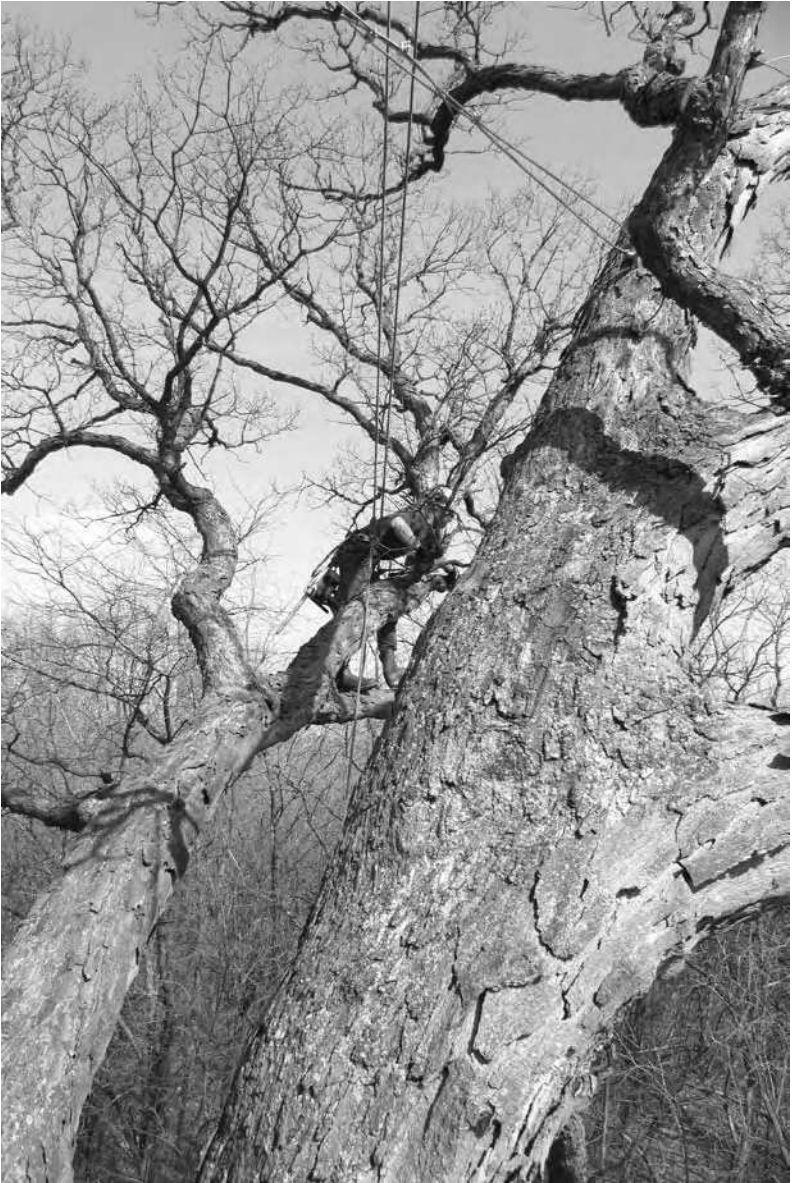
Installing reinforcing cables on one of the major side limbs, high in the crown.
