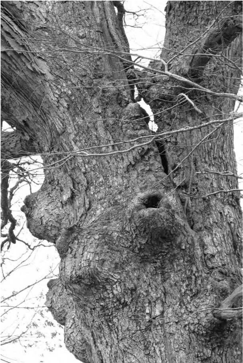
The main fork of the trunk, showing the split that caused the project to be undertaken.
