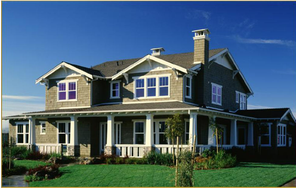
Predominant gable elements with heavy ornamental detailing at gables and a full porch
