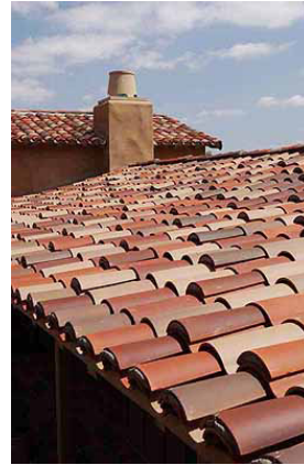
Roofing in a subtle terra cotta blend
