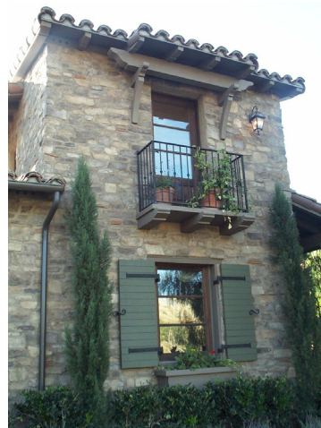
Balcony with wrought iron railing and exposed rafter tails
