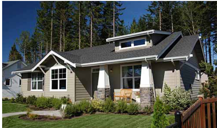
Battered columns resting on masonry piers at porch
