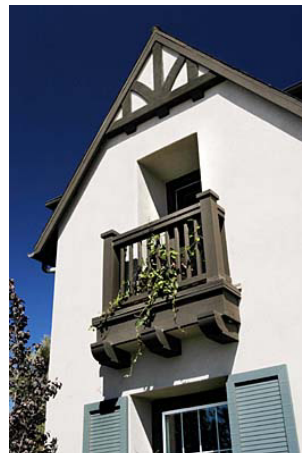
Wood trim at gable end
