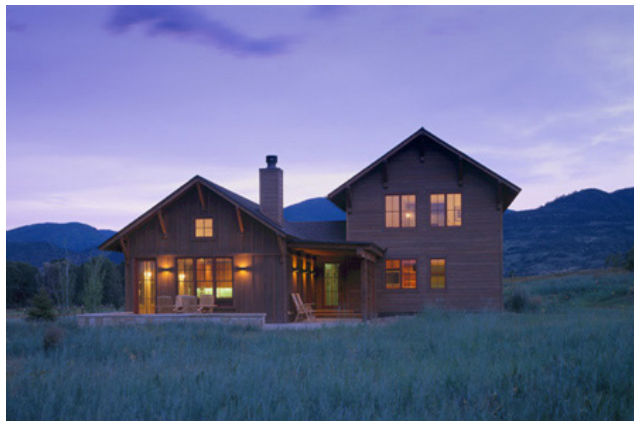
Simple gable forms with heavy wood detailing at gables
