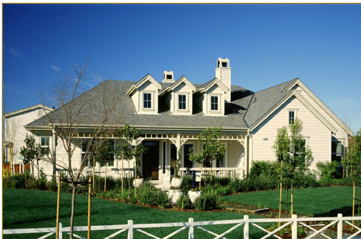
Dormer windows and predominant porch
