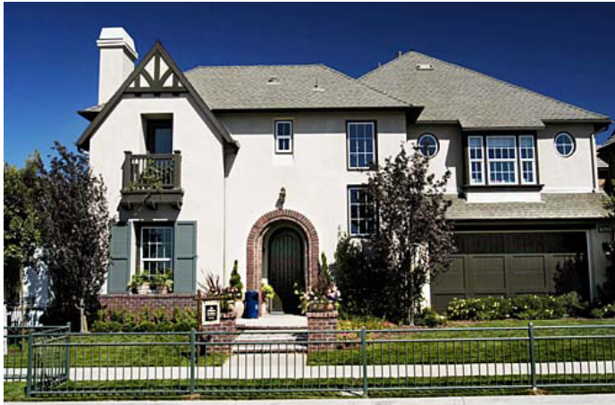
Lowered roof plate at second floor and masonry accents
