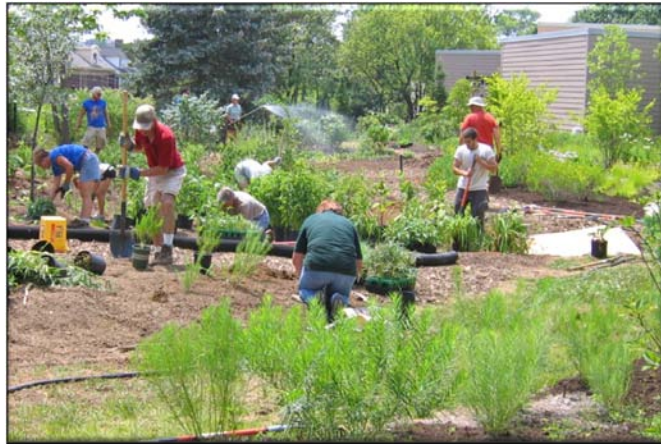
Fig. C-20: Planting a rain garden Photo by Dave Dyke
