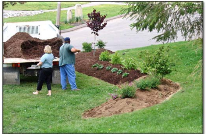
Fig. B-8: Mulching CIP with 2" of shredded hardwood mulch Photo by Dave Dyke
