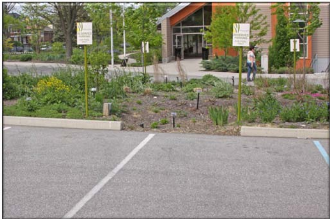
Fig. C-8: Curb cut allowing water to flow from a parking lot into a rain garden Photo by Joe Boggs
