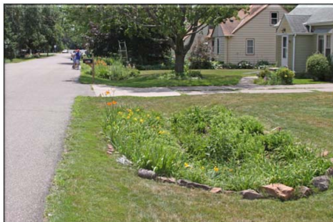
Fig. C-1: Series of residential rain garden installations to infiltrate water runoff from a street
