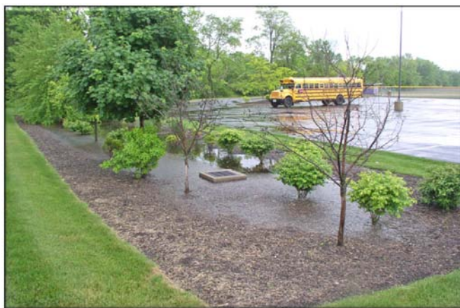
Fig. A-1: Elevated overflow drain in rain garden Photo by Dan Ross, USDA NRCS
