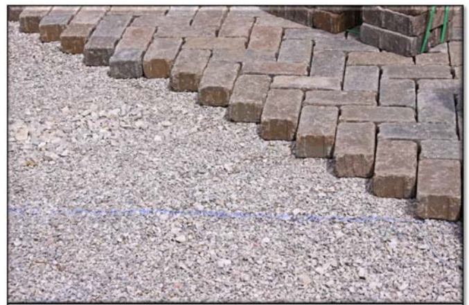
Fig. 5: Pervious paver installation to enhance water infiltration Photo by Joe Boggs
