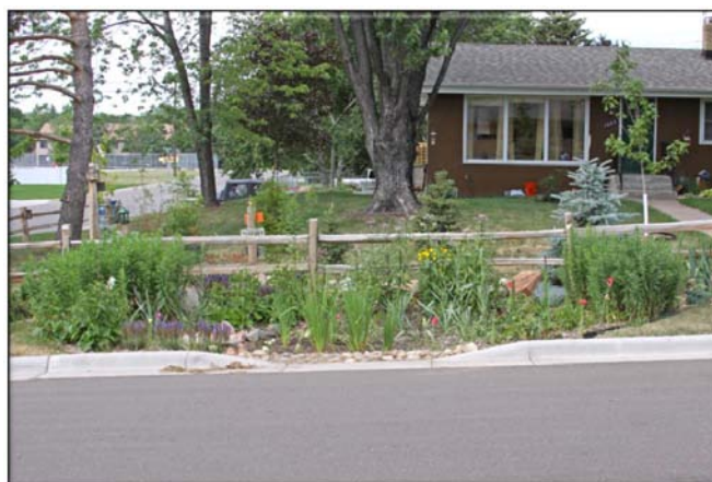
Fig. C-2: Residential rain garden installation to reduce water runoff from a street
