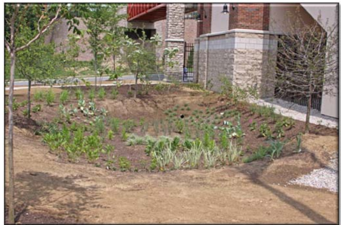
Fig. C-21: Completed newly installed rain garden Photo by Joe Boggs
