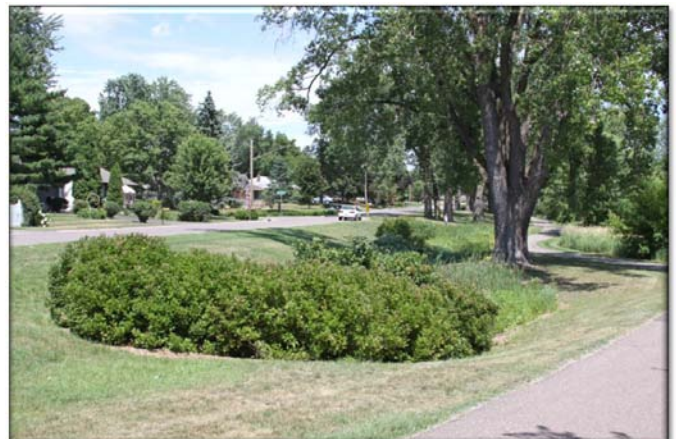
Fig. A-5: Rain gardens using shrubs and incorporating established trees for water uptake and removal Photo by Joe Boggs
