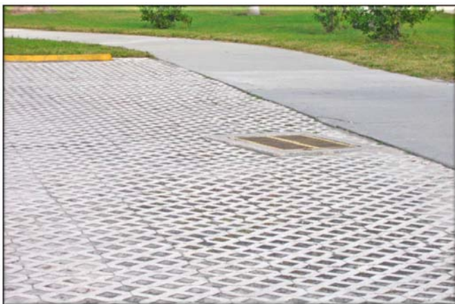
Fig. 4: Pervious pavers in a parking lot Photo by Dave Dyke
