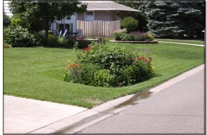
Fig. A-3: Residential rain gardens installation to infiltrate water runoff from a street Photo by Joe Boggs
