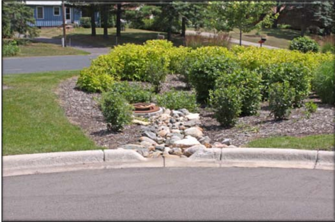
Fig. A-2: Parking lot curb cut-out, stones to slow water movement, and elevated overflow drain Photo by Joe Boggs
