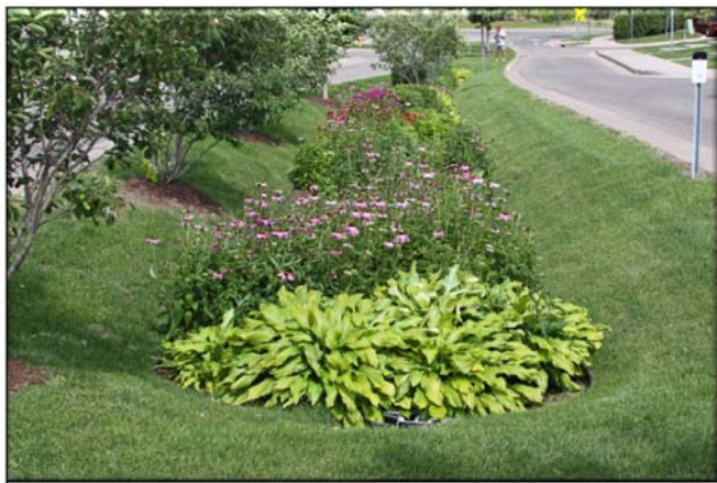
Fig. A-4: Community rain gardens installation to infiltrate water runoff from streets Photo by Joe Boggs
