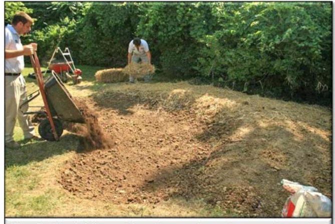
Fig. C-14: Adding soil and amendments to a rain garden Photo by Bill Shuster, USEPA-RD
