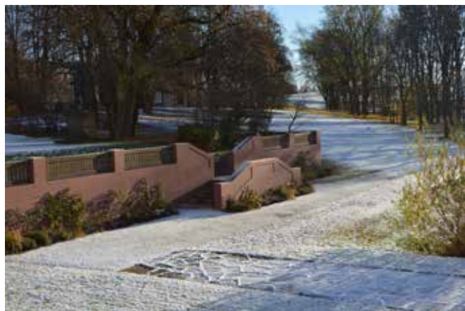
■ Fig. 1. The Hirsch stairs is a key element in Moens design for the University Park. They were removed in the 1960's and reconstructed 2016-17. (Photo: Bjørn Anders Fredriksen, 2017)
