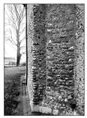
Photograph 2. North-west corner of the nave where it abuts onto the tower, showing the flint quoins of the Saxon wall of the nave and the fillet of brick and flint bridging the corner between the nave and the tower.
