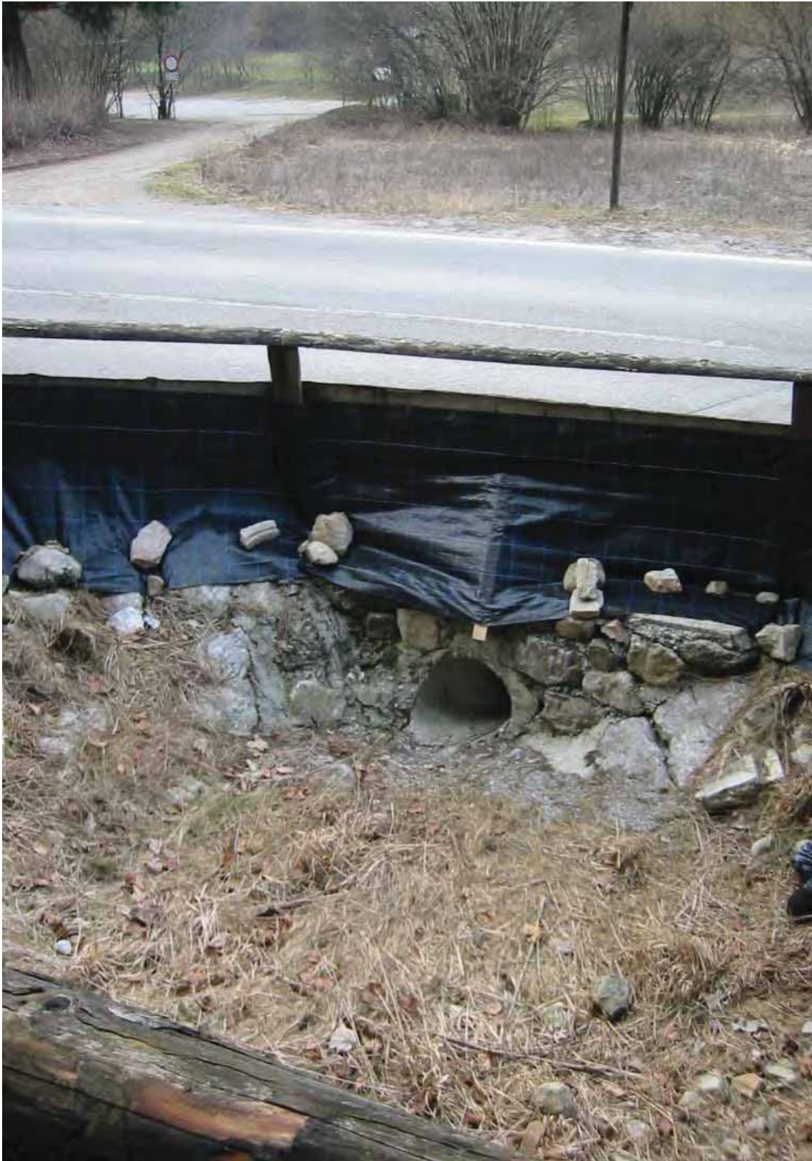
Tunnels under roads to encourage the migration of amphibians, at the Fiaavè peat bog
