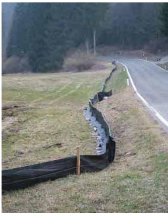
Barriers to protect spring migration by amphibians along roads, at the Fiaavè peat bog
