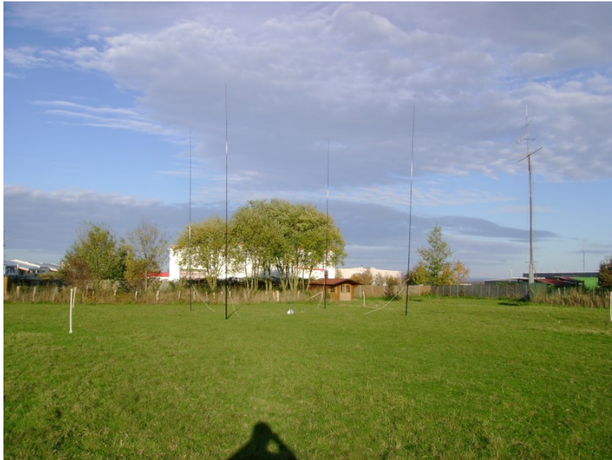
Figure 6.1 40m 4-square with one elevated-radial at DF0AT
