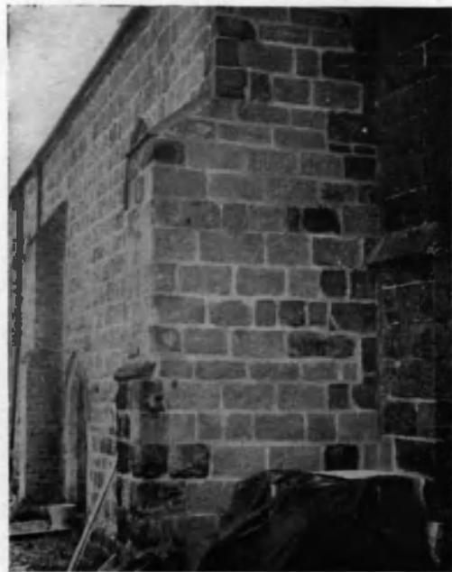
MALTBY CHURCH, LINCS., 1940. After Repair in 1940.
