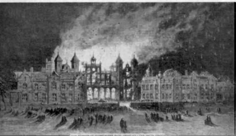
Fire at Capesthorpe, 1861.
