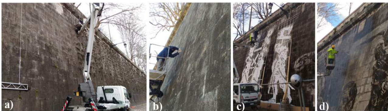
Fig. 1 Different phases of the rural vegetation removal (a-b) and cleaning for the realization the artistic work (c-d).
