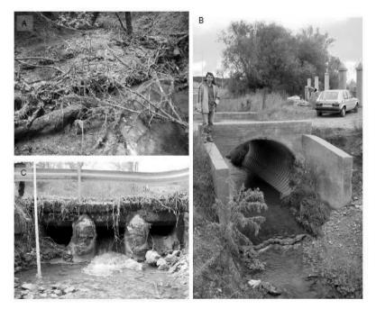
Fig. 1. Examples of common culvert barriers (photos J. García Molinos): (A) large volumes of sediment and debris accumulated upstream of an undersized culvert, (B) poorly graded corrugated pipe culvert creating a depth barrier, and (C) multibox culvert with perched outlet.
