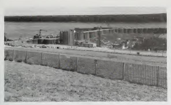
**Figure 13** Lock cofferdam at the Olmsted Locks and Dam Project. The cofferdam is used to hold back the Ohio River during construction of the locks. Approximately 41 acres are within the coffered area (photo by Wayne T. Frankie).
