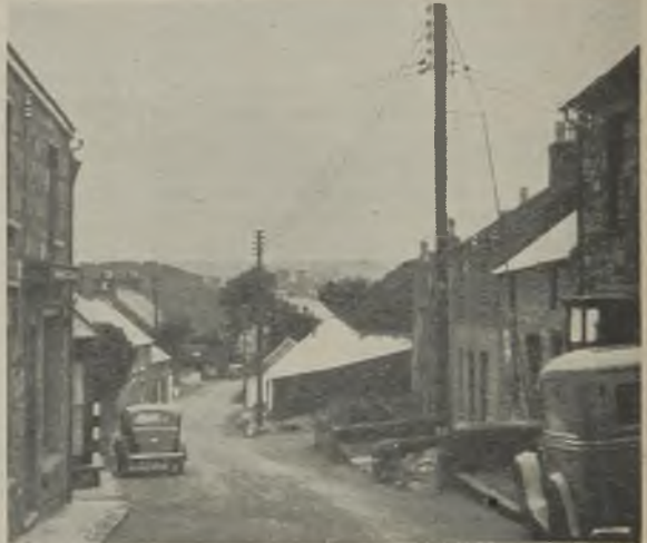
Low-voltage overhead mains at Newport, Pembrokeshire
