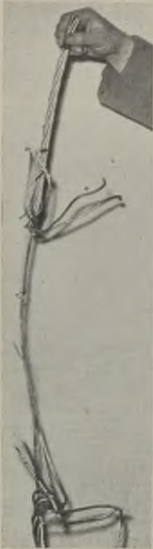
A piece of 33-kV cable which for 24 hours carried the whole of the power for the Dover district through the steel suspension core, after the outside aluminium conductor strands had been severed by a fragment of shell during a raid
