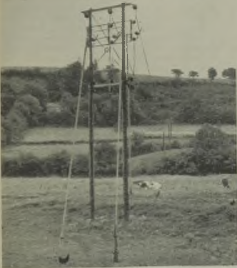
Top: A typical section of single-circuit 22-kV overhead line Right: 25-kVA, single-phase, pole-mounted transformer supplying Llanfihangel-ar-Arth Below: 22-kV line to supply Llandyssul (under construction)
