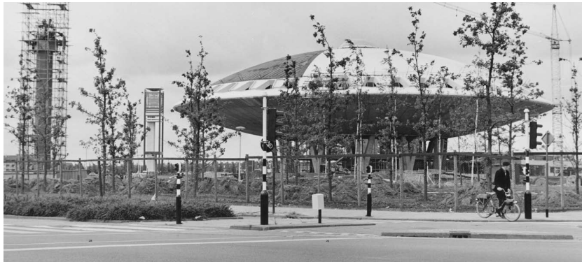
Figure 11. Two kinds of communications towers under construction. (Source: Hendriks, 28-29.)
