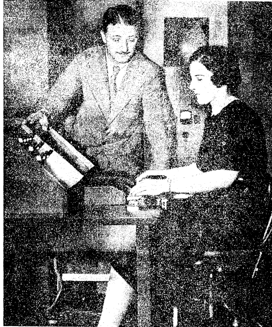
Figure 7. S. S. A. Watkins and Helen Amelia Harper give one of the first public demonstrations of the Voder at the Franklin Institute in Philadelphia on January 5, 1939. (Associated Press) (“Machine Talks in 23 Human Voice Sounds,” Chicago Daily Tribune , January 6, 1939, 2).
